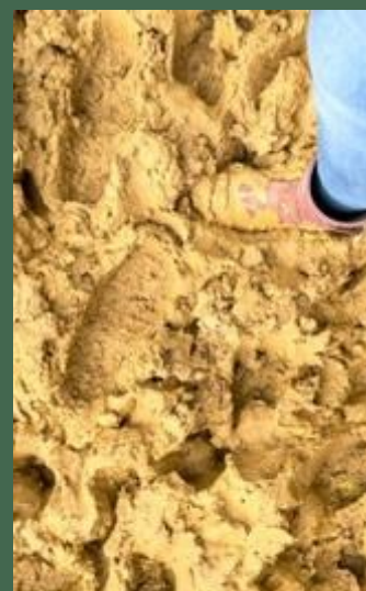
Left - David Ffrench and Patrick Hickey assessing the fourth test site displayed a small percentage of marl, which is required to form a compatible mix. Middle - Cattle treading the mortar, Right - Treading by foot.
