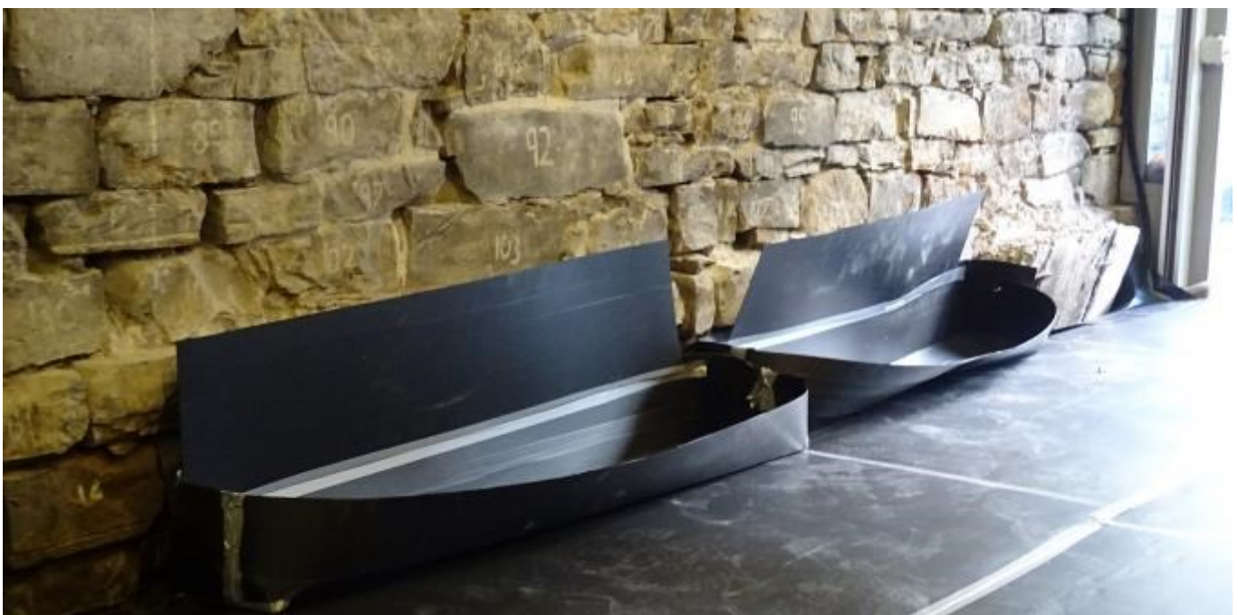
Material from the raked out joints was collected and processed.
