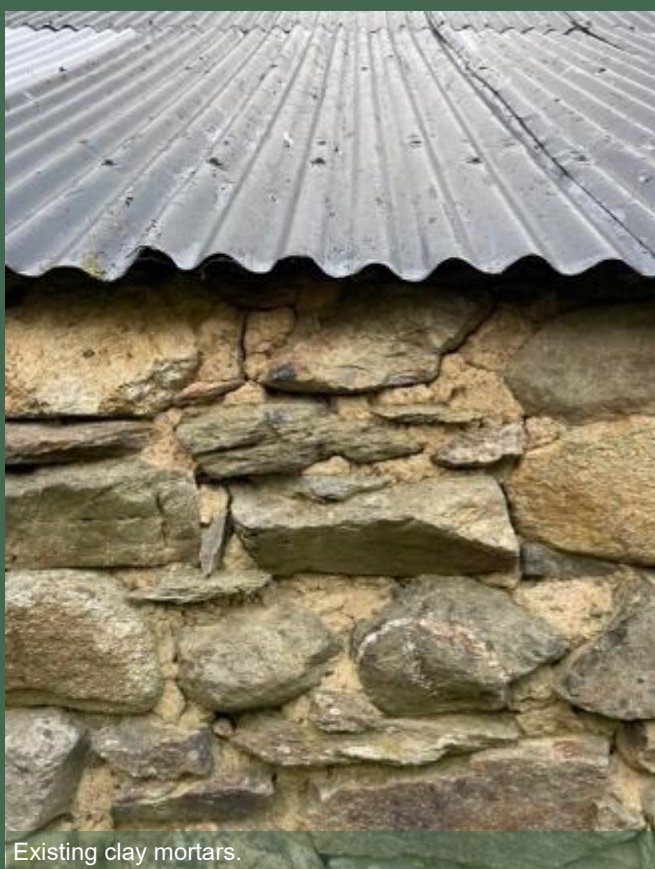
Eroded tempered clay exposing aggregate.
