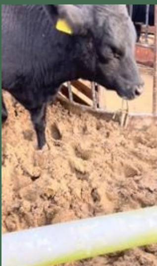
Left - David Ffrench and Patrick Hickey assessing the fourth test site displayed a small percentage of marl, which is required to form a compatible mix. Middle - Cattle treading the mortar, Right - Treading by foot.
