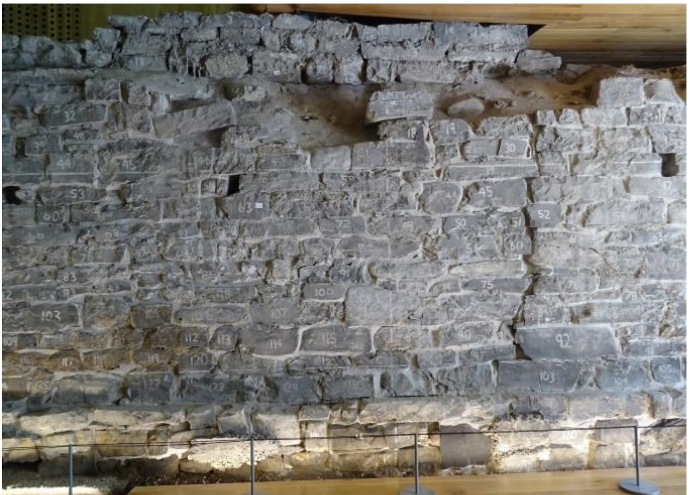
Dublin city wall following completion of the works.
