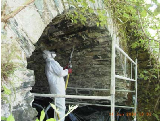
Figure 5: Repointing using sprayed mortar
