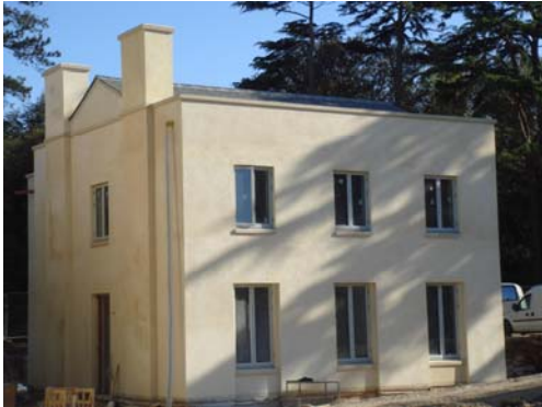
New Building, Lime used at all stages of construction.
